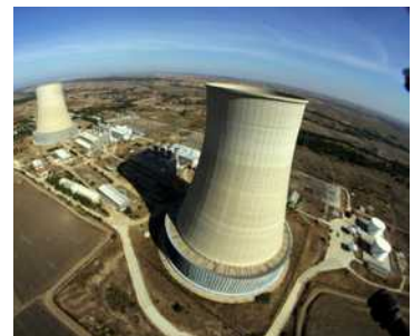
Power Plant Chargers
